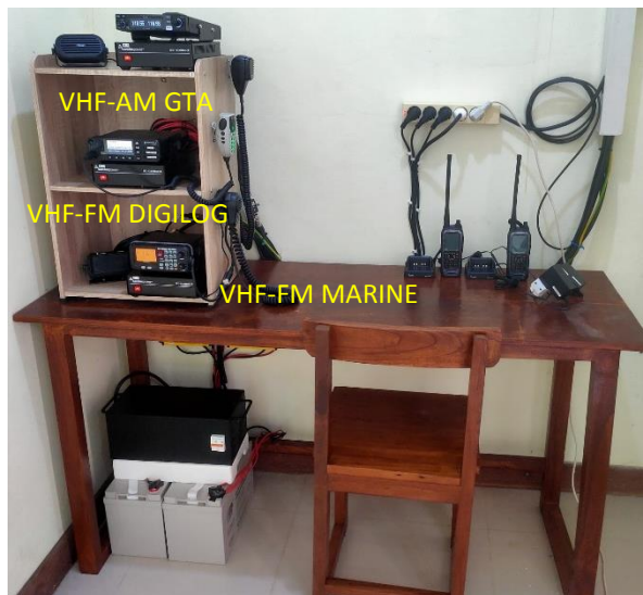
Gambar 21 Base Communication System USPP Bangsal dan USPP Mandalika
